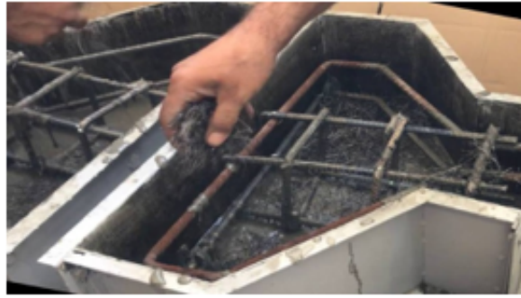
(a) Manual distribution of steel fibers
