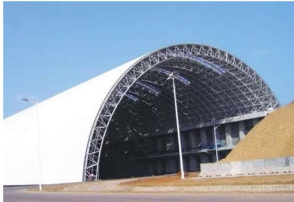
Gambar 1. Space Truss Type Barrel Vaults
